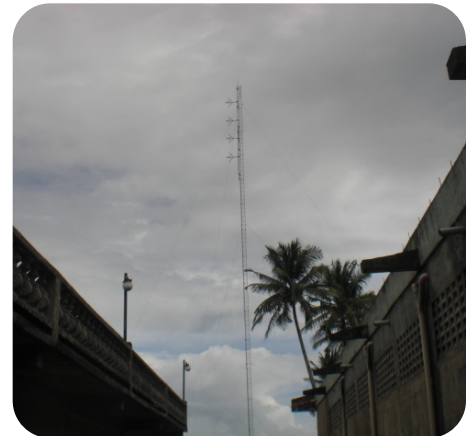
150' Tower in San Jose, Samar The entire tower erected with the 4 bay antenna that reaches over 320 miles to the north
